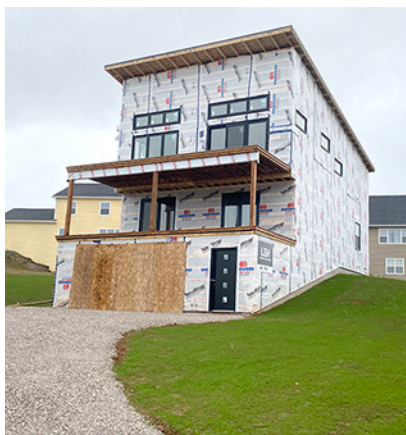
A new build by R. Seegers Construction.
