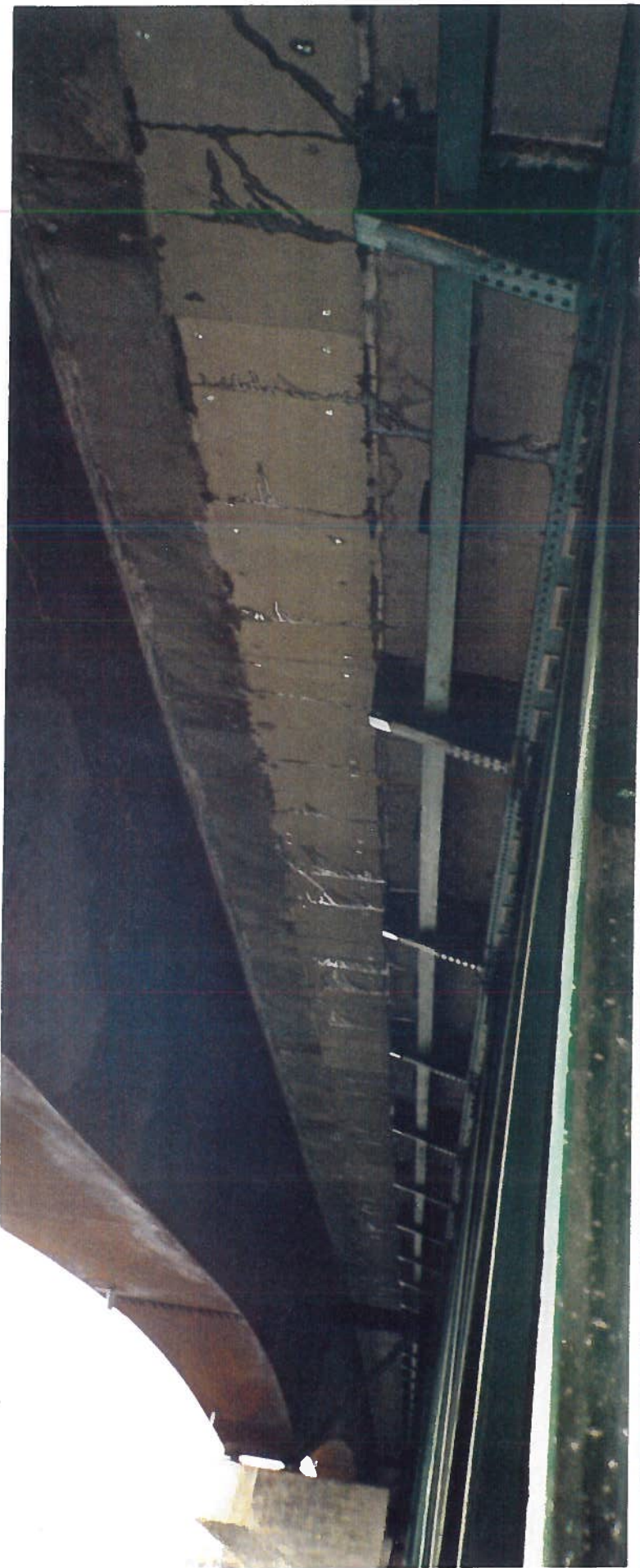
Cracks in in-fill strips.
