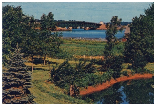
Photo 1.3: Hillsborough Bridge before 1996 Upgrades
