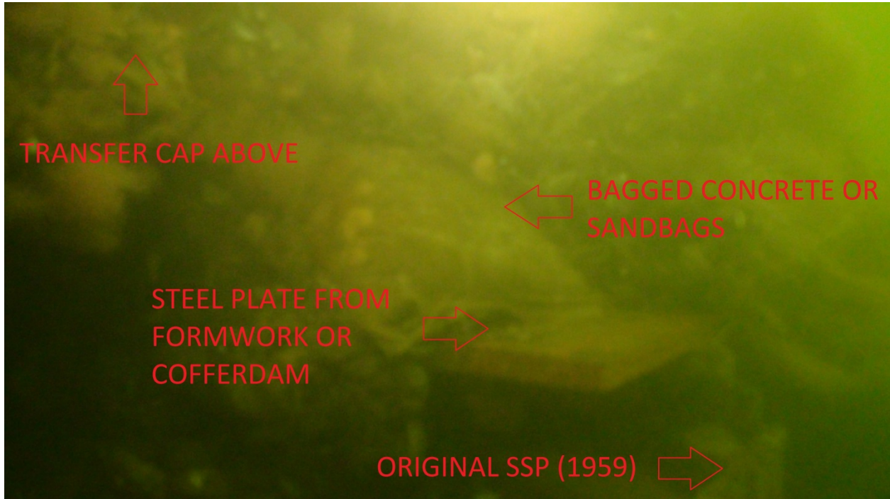
Photo 6: Additional formwork at the base of transfer cap.
