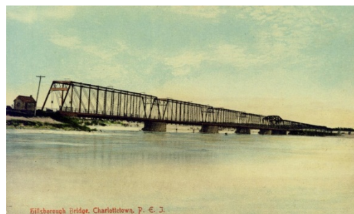
Photo 1.2: Old Hillsborough Bridge 1907
