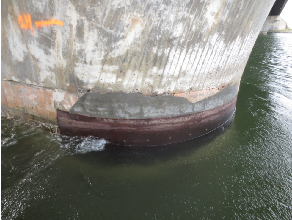
Photo 11: Repair of concrete above ice shields.
