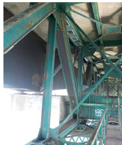
Photo 3.9: Limited View of Top Chord from Access Platform
