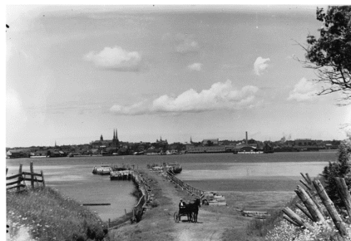
Photo 1.1: Bridge Site before 1905
