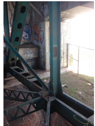
Photo 3.6: Coupon Taken from Vertical at U37-L37 Right
