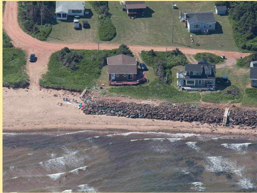
Figure 4.3: Example of armouring (Photo credit: Don Jardine)
