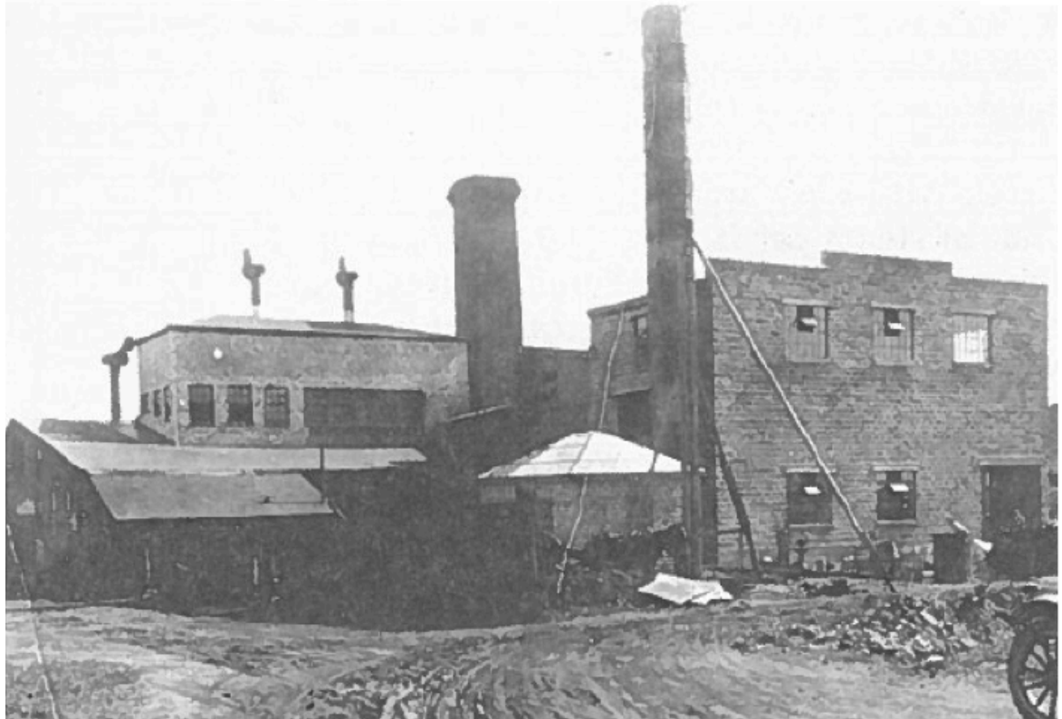
Figure F.1: Exterior View of Maritime Electric Company Plant in Charlottetown, 1926.
