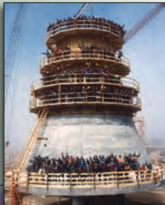
Left: Workers on a pier shaft in the Borden fabrication yard.
