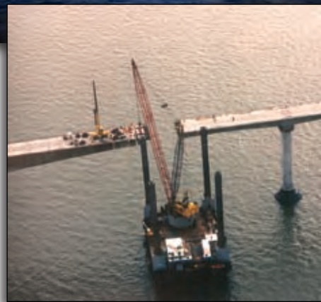
Right: Oct. 22, 1996, main bridge meets approach bridge.
