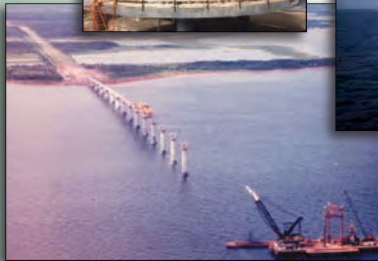
Above: West approach bridge.
