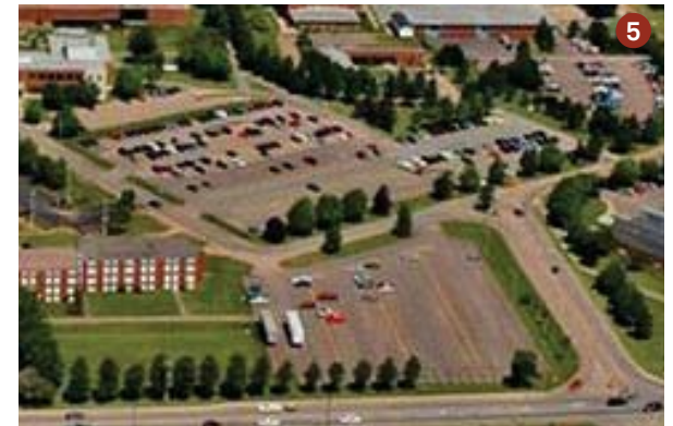
Parking Lot Improvements
