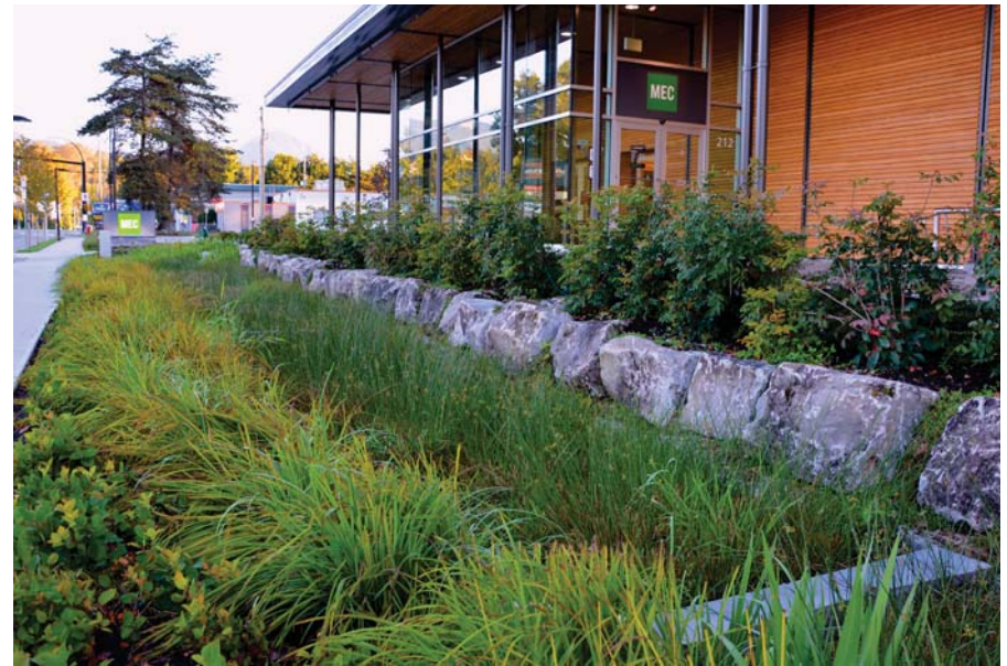
Rain gardens accept stormwater runoff from nearby paved areas
