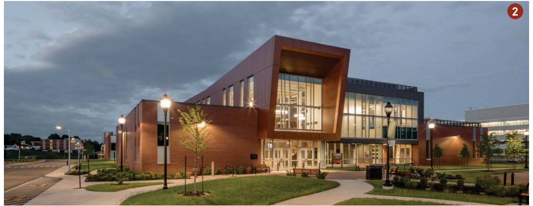
Sustainable Design Engineering Building
