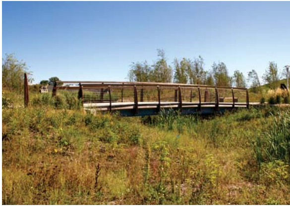
Bridges and boardwalks can be used in the Vale Nature Area to manage topography and wetlands
