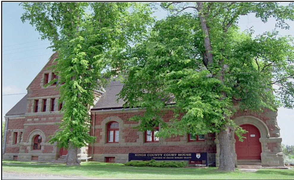
Three Rivers has many buildings of architectural and historical significance including Kings County Court House, located in Georgetown.
